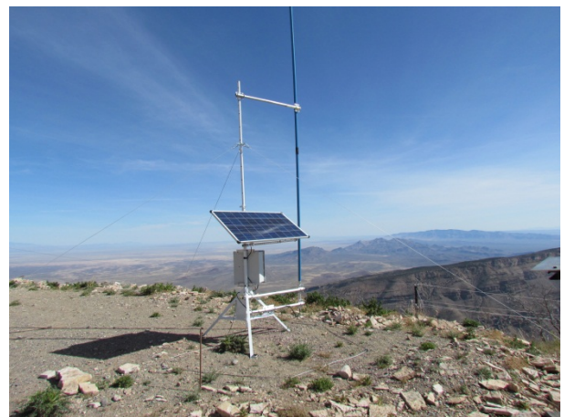
Figure 6: NGBPS C2 Repeater Station
