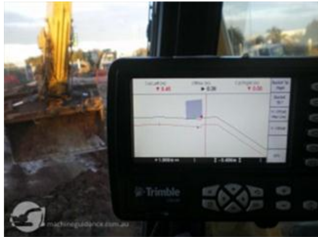
Figure 5 3D Machine Guidance Interface setup on excavator
