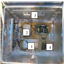
Figure 5 Internal Box Configuration1. LocataLite2. Meteorological Sensor3. Amplifier4. Power Supply
