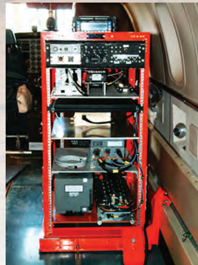
Typical Rack- Mounted System
